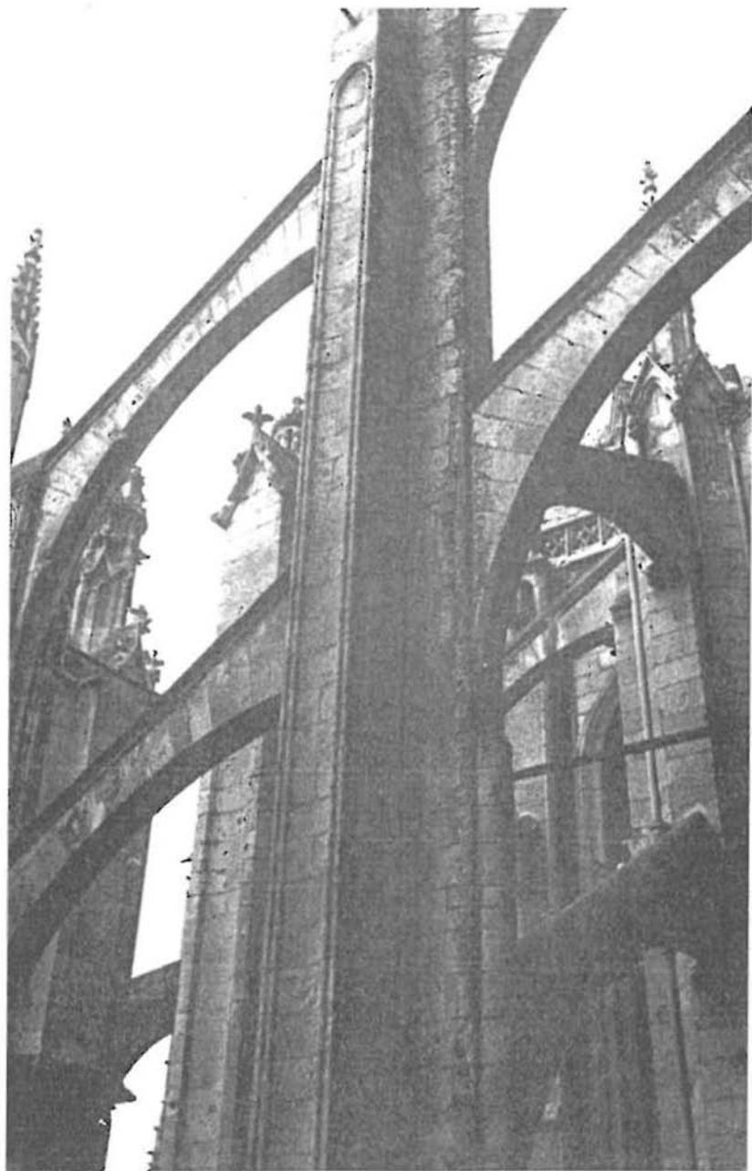
FIGURE 9. *Intermediary flying buttress upright, bay 7, south side.*
