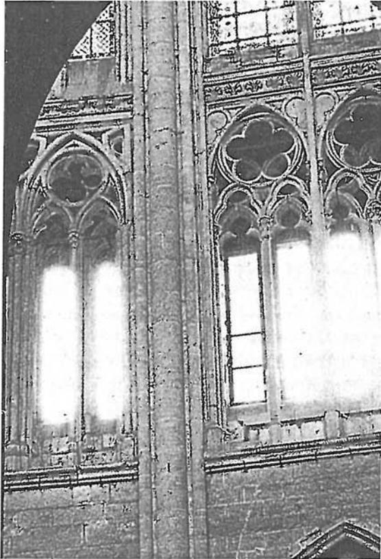
FIGURE 2. *Detail of the triforium at bay 8 on the north side, showing the transition from pre-collapse to post-collapse tracery.*
