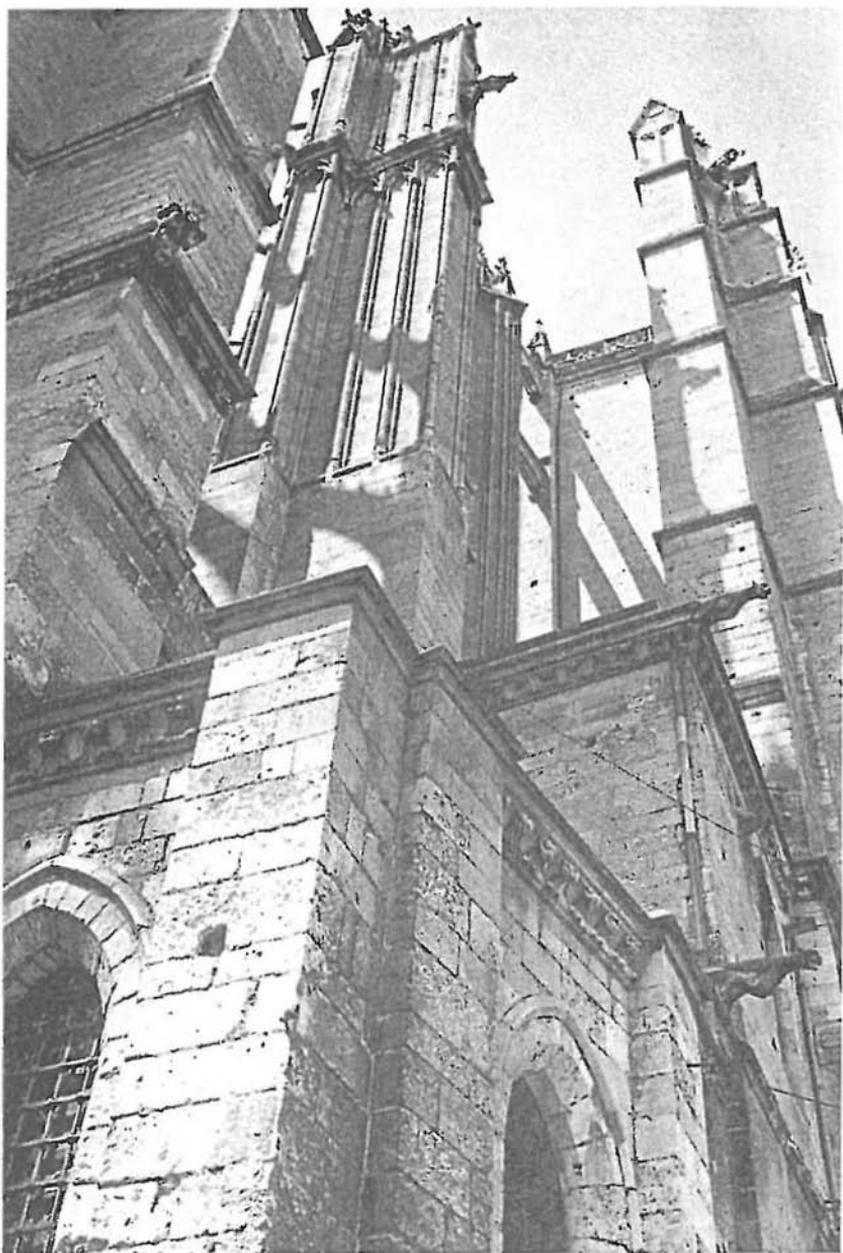
FIGURE 7. *Outer upright of flying buttress, bay 7, north side.*
