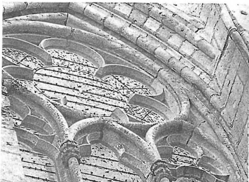
FIGURE 3. *Detail of re-used tracery in clerestory window.*
