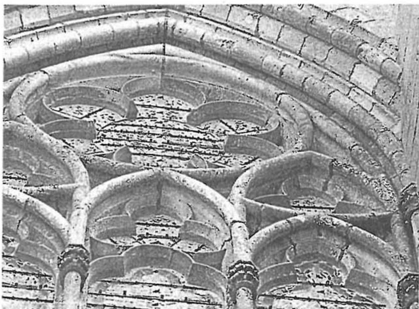
FIGURE 4. *Detail of tracery made in the campaigns of repair after the collapse.*
