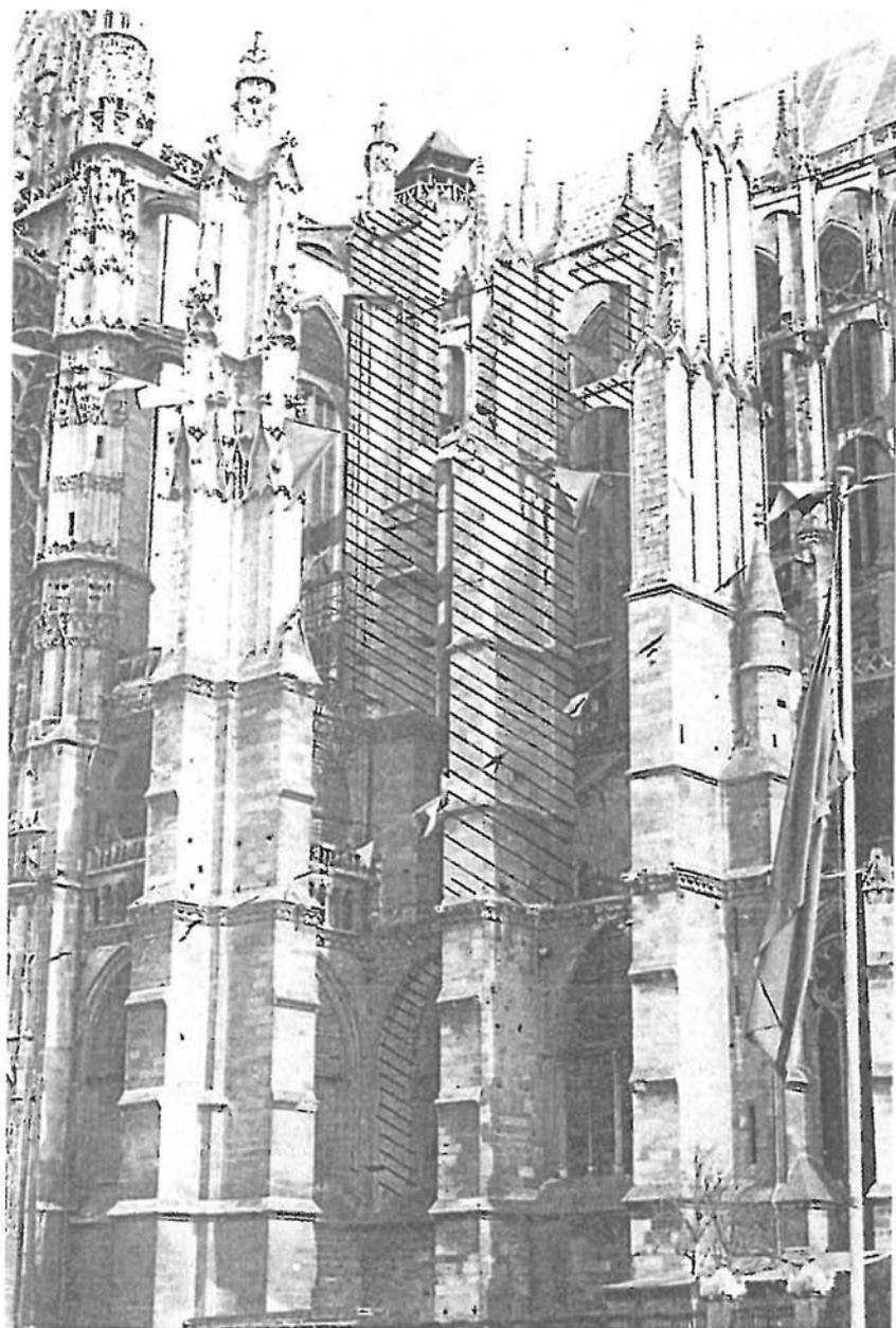
FIGURE 10. *General view of the south side of the choir. Cross-hatching indicates parts rebuilt after the 1284 collapse.*
